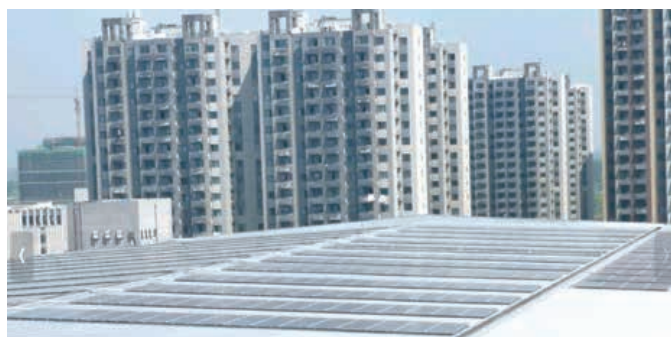
Photovoltaic power station in Hefei industrial park
