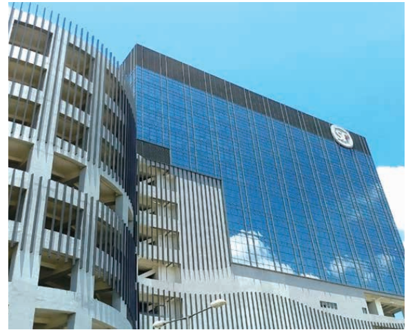
SF Holding Hong Kong industrial park
