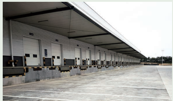
Permeable Concrete Construction in Nanning Park
