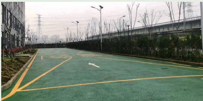
Permeable Concrete Construction in Hangzhou Park
